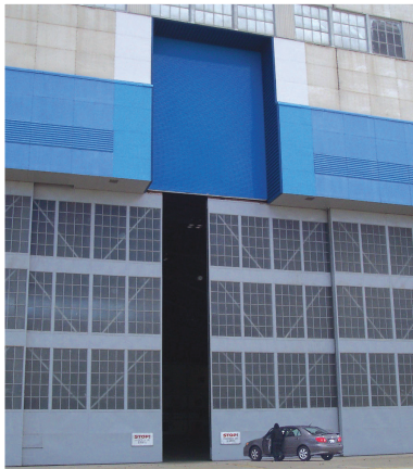
Tail cut out above the massive doors allows the 747SP's 65-foot high vertical stabilizer to enter the hangar. It is one of several major investments by NASA to tailor N211 for SOFIA .
