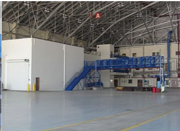
The skywalk will afford access to the plane's port side; next to it (and also new) are two high-bay rooms for mirror stripping and mirror coating. Yellow lines in foreground mark the center taxi line for the aircraft.
